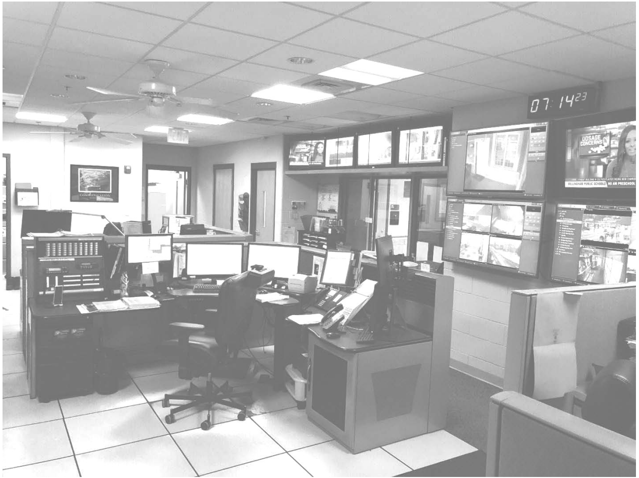
Hopkinton Public Safety Communications Center
